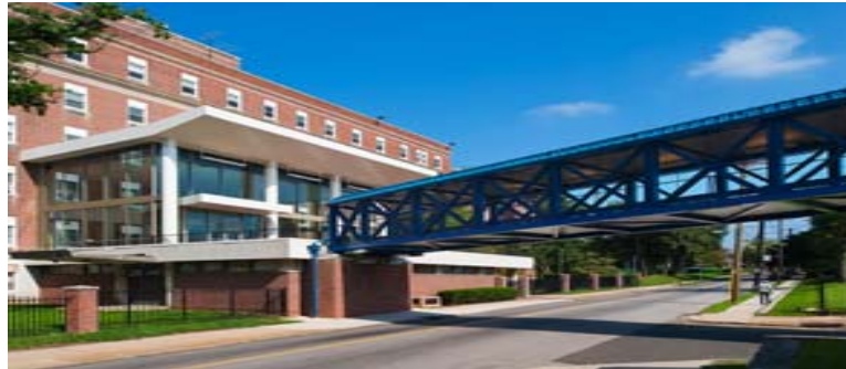
Figure 6.3 The Bridge From the Main Campus.
